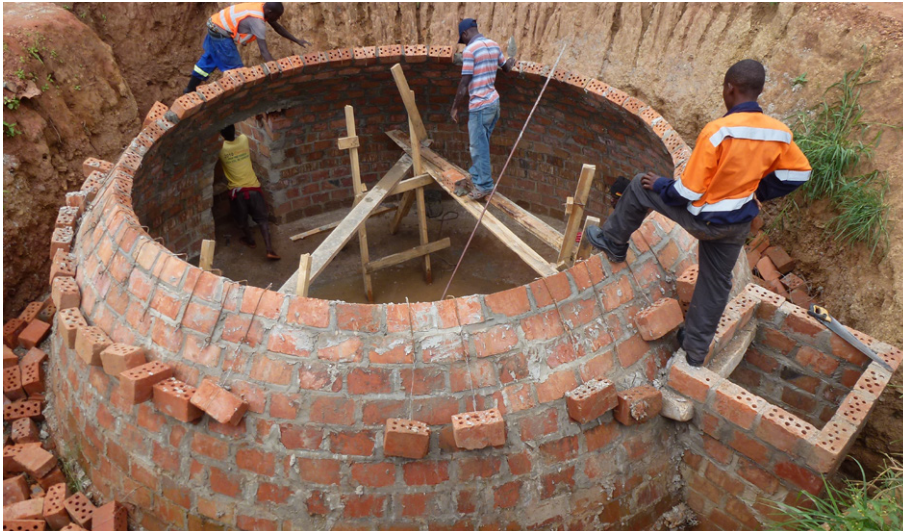
Image: FSM transfer station under construction in Chazanga, Lusaka
